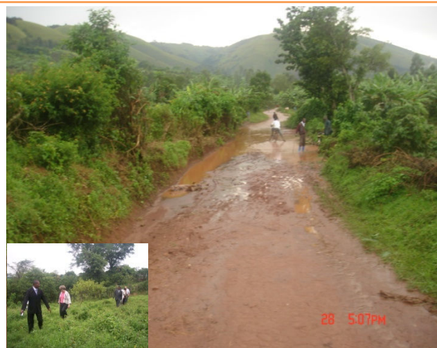
Some Infrastructural Hindrances' to Couple Visits
